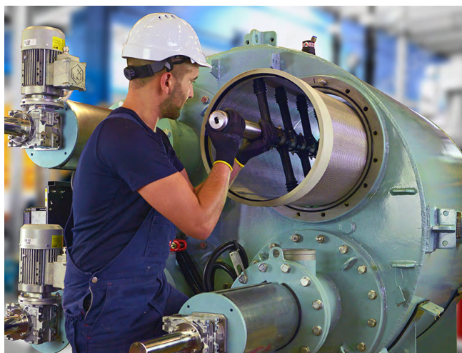
Installing our patented nozzlex screen cleaning technology within a BSE Multi-Screen filter.
