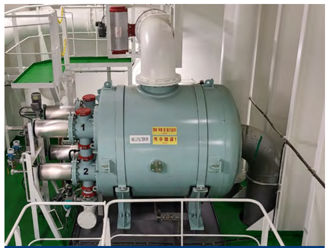
Our BallastSafe filters are modular and can be oriented in any direction to fit any installation.
