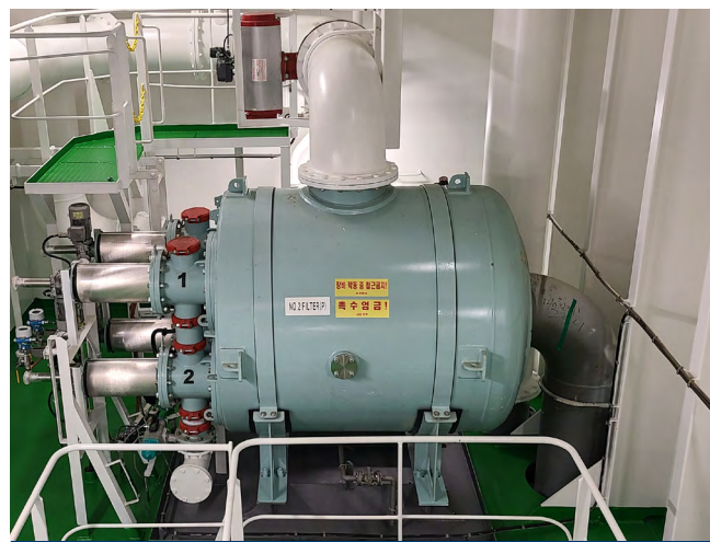
Our BallastSafe filters are modular and can be oriented in any direction to fit any installation.
